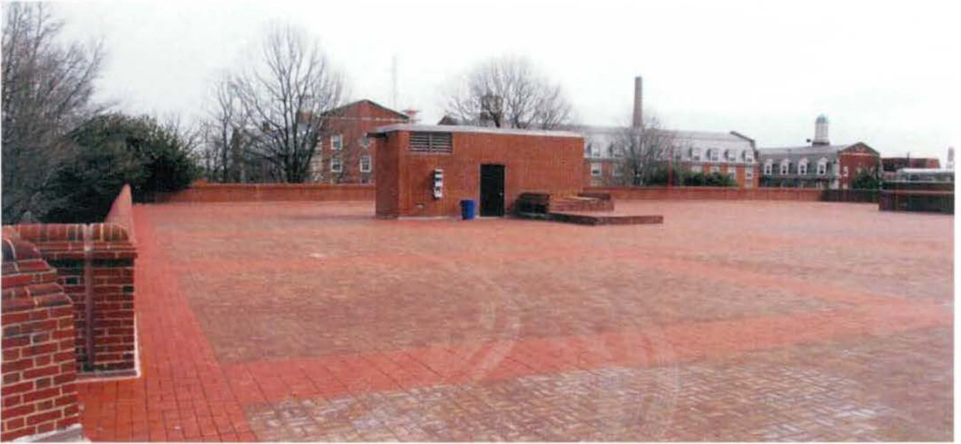
Photo 6-3: View of existing roof of Undergraduate Library
